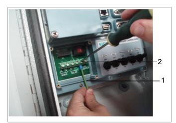
Fig. 51 Earth wire connection in terminal block
