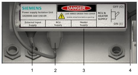
Fig. 10 Power Supply Isolation Unit
