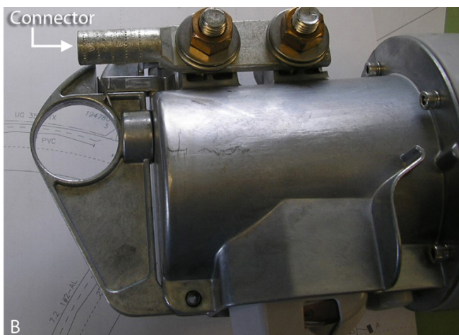
Figure 8—Two-Hole Lug Connector (SI# 4670256)
